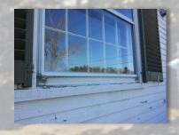
**Windows:** Several of the 10 -foot-tall windows in the sanctuary are not weather tight and need major energy efficient repairs both inside and out.
